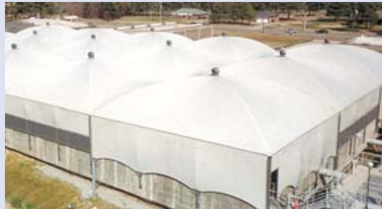
Water Treatment Facility; Chesapeake, VA
