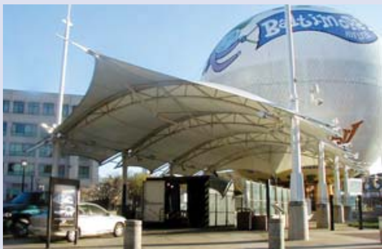
Shot Tower/Marketplace Metro Station Entrance; Baltimore, MD
