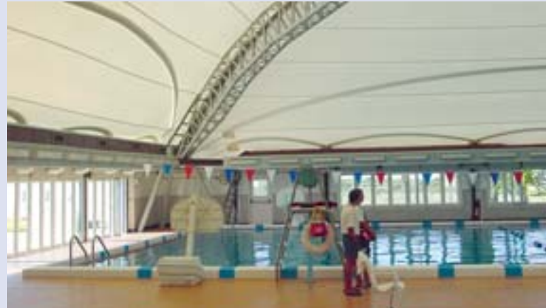
Pool Enclosure; Rota, Spain
