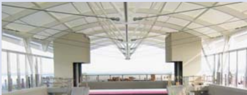
Lightwell; Raleigh-Durham International Airport
