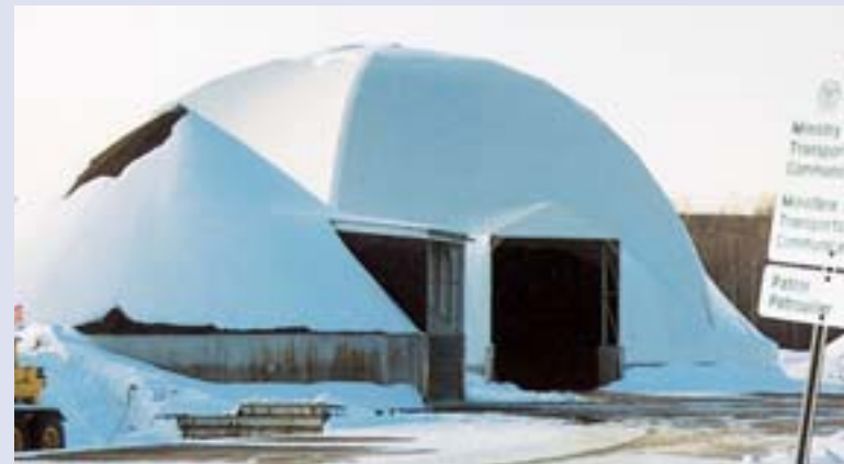
Sand/Salt Storage; Ontario, Canada
